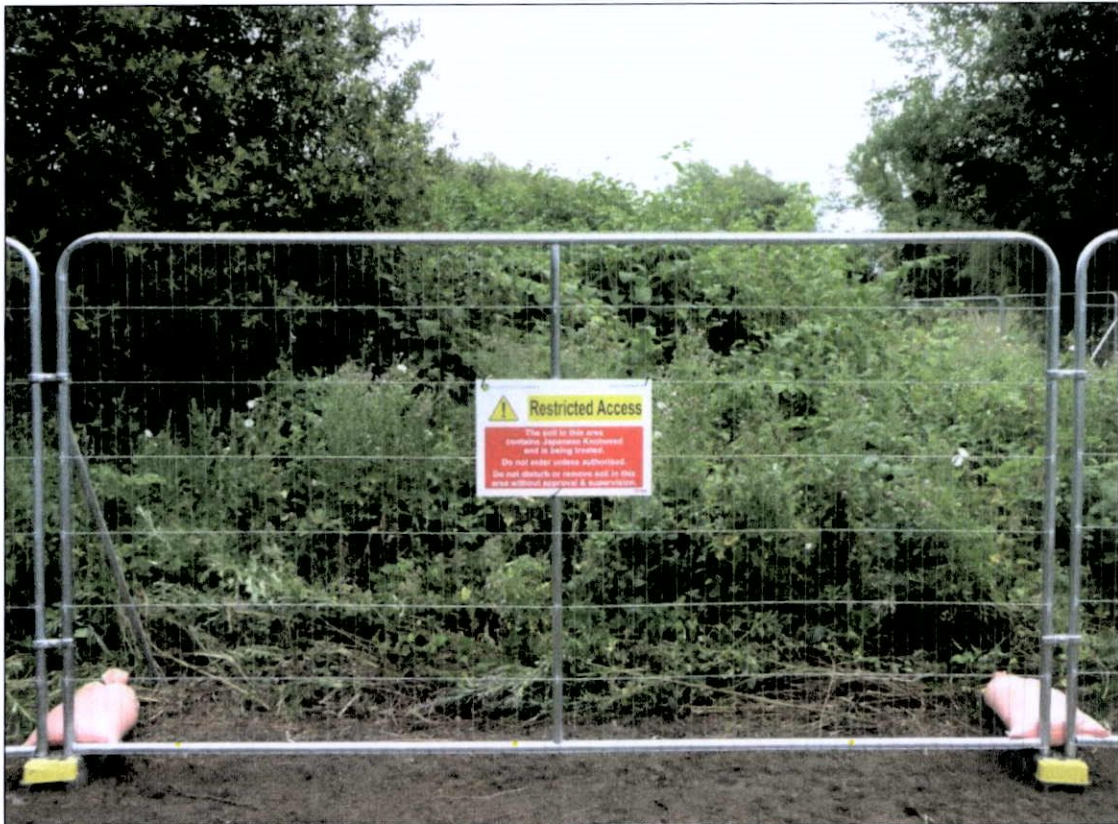
SAMPLE FENCING 2 – HEAVY DUTY HERRAS FENCING
