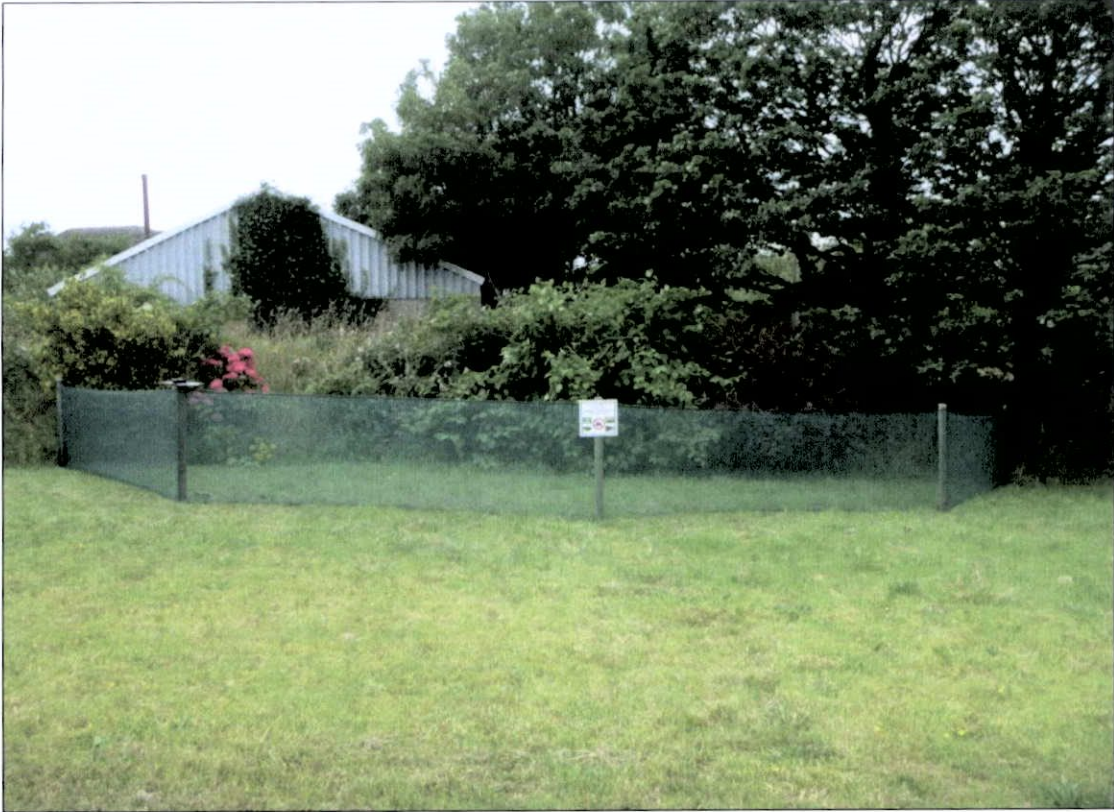
SAMPLE FENCING 1 – POST AND WOVEN MESH FENCING
